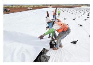
Rain cap: In this 2011 file photo, workers with Black Construction and Northwest Linings pull sheets of rain cap to cover a cell at the Layon landfill. Pacific Daily News file photo
