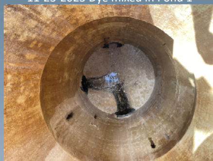
11-25-2023 Checking for dye in manhole
